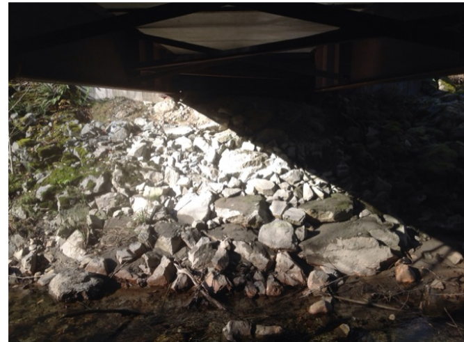
Right Bank Abutment when facing downstream
