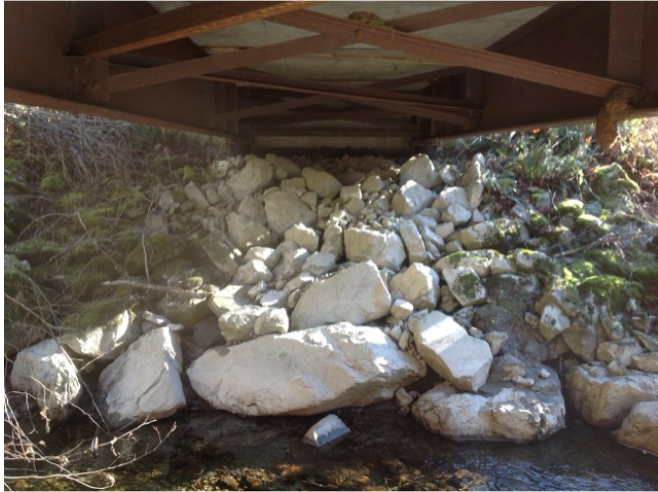
Left Bank Abutment when facing downstream
